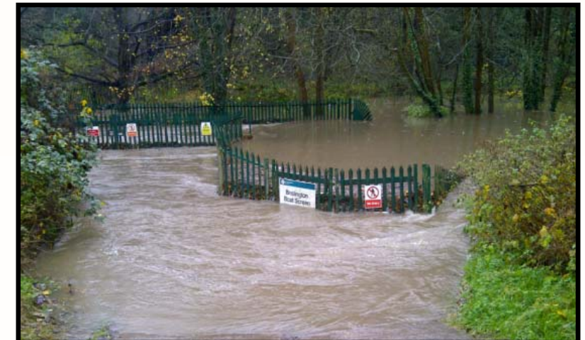
Screen blocked during flood
